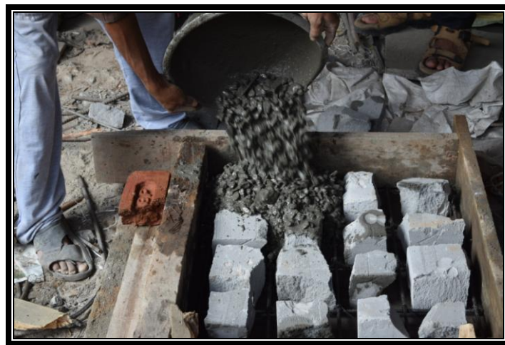
Figure 3. Casting of slab.
