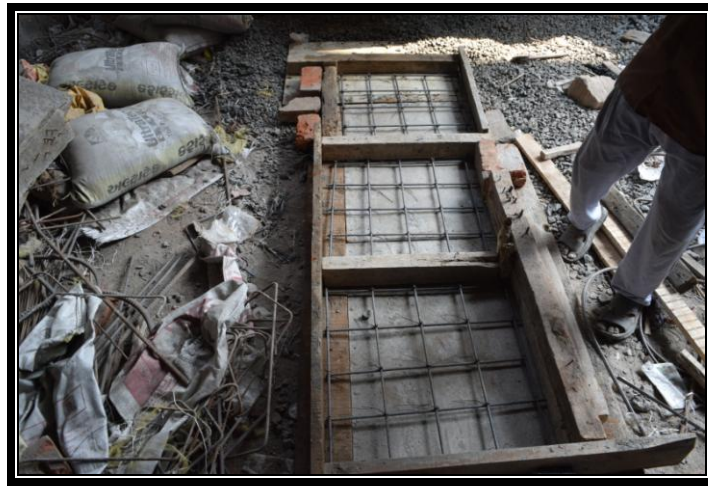
Figure 2. Reinforcement for slabs.
