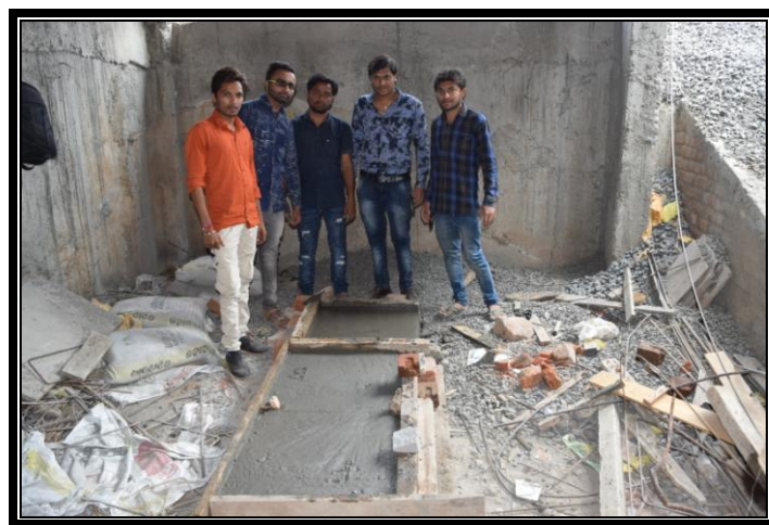
Figure 4. Casting of slab.
