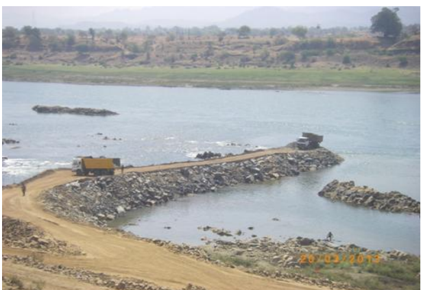
Figure 4. Under construction Garudeshwar weir site
