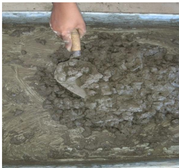
Figure 2. Mixing of SCBA in Concrete
