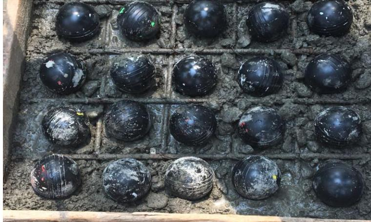
Fig 1: Bubble deck block
