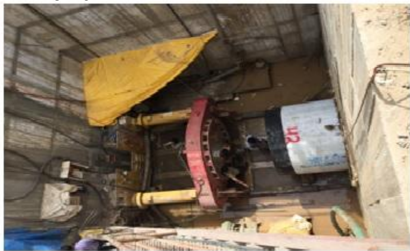
Fig.4 Pipe Jacking (Pipe-42) at R.C Dutt Road, Vadodara.
