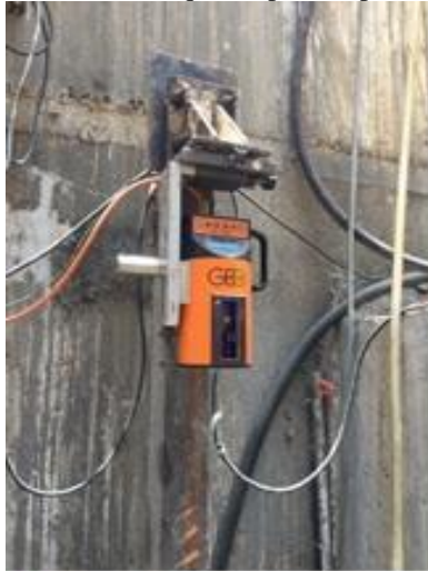
Fig.3 Laser alignment Process at R.C Dutt Road, Vadodara.
