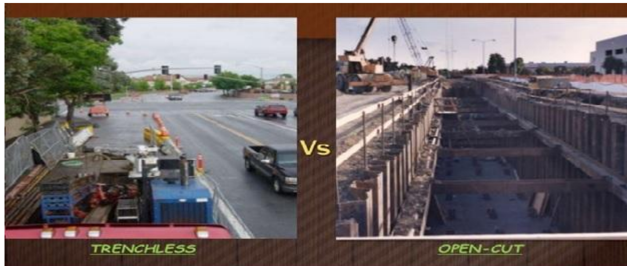
Fig.2 Comparision with Open Cut Conventional Method
