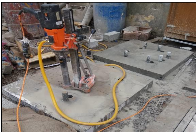
Figure 8. drilling cores from slabs
