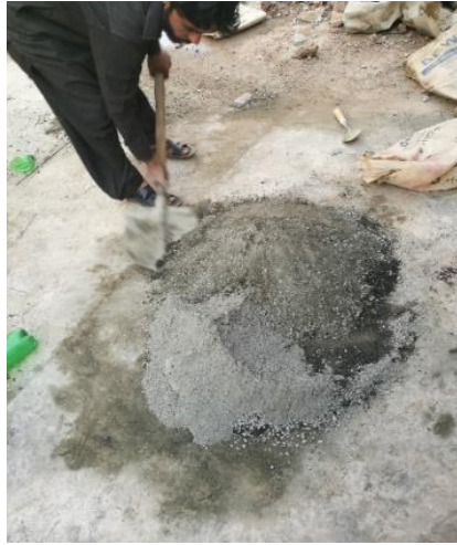
Figure 13. Material Mixing through Shovel
