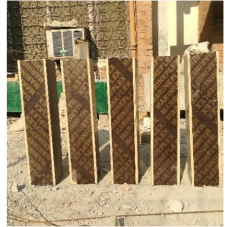
Figure 9. Formwork for Models
