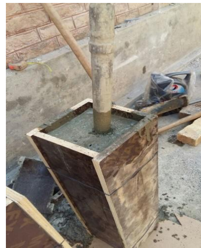
Figure 16. Vibration through Concrete Mixture
