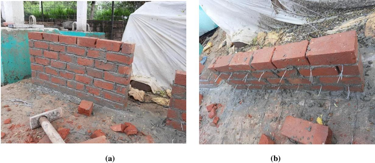
**Figure 3:** (a) Preparation of the unreinforced masonry prism (b) Preparation of panel reinforced with wire mesh
