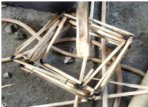
Fig. (d): Bamboo Stirrups Fig. (e): Gas used for made up of stirrups
