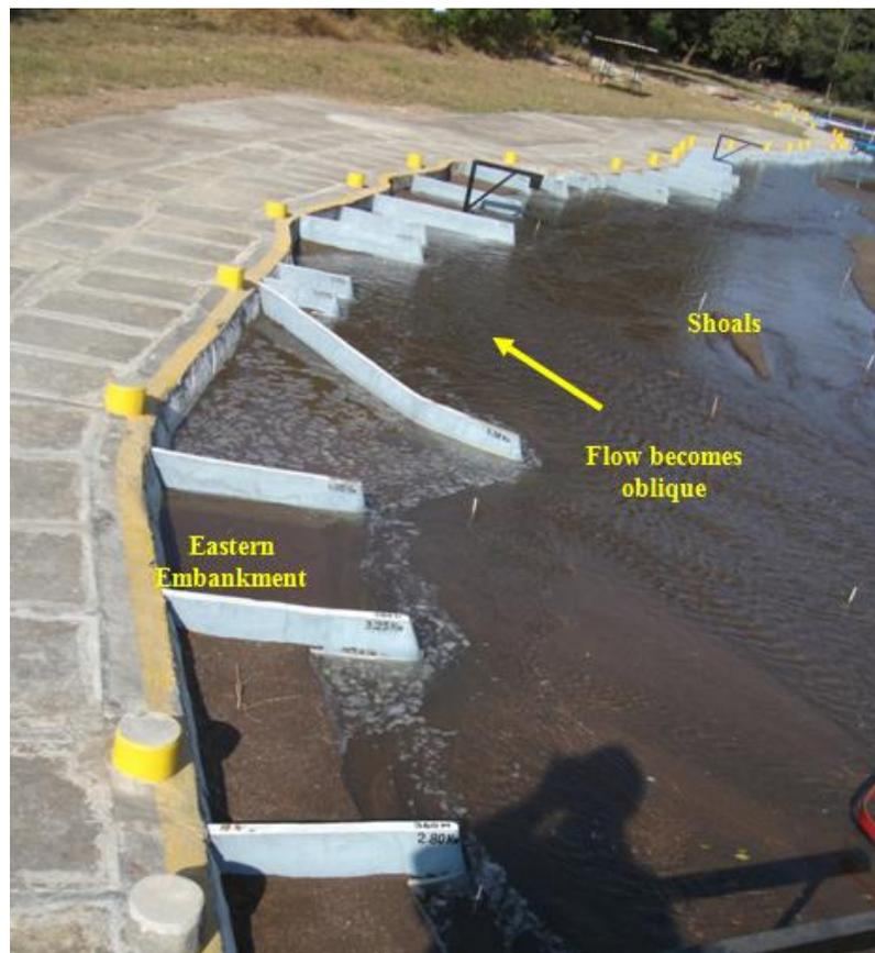
**Figure 14** Close view of flood embankment ( $Q = 15,586 \text{ m}^3/\text{s}$ )
