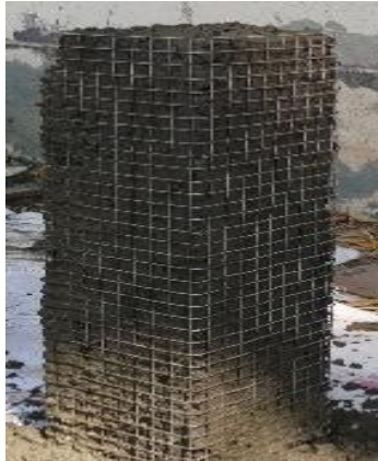
Fig. 3 wrapping column using single layer wire mesh
