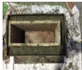
Shuttering and casting of ferry boat
