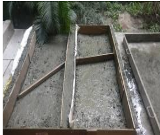
Figure 5 :- Complete casting Normal Concrete for (MSA)Slab
