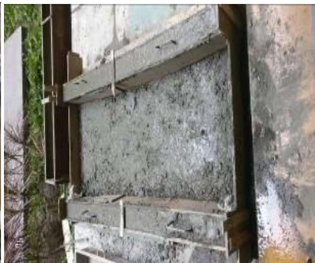
Figure 9 :- Complete casting of normal concrete in (MSB) Slab
