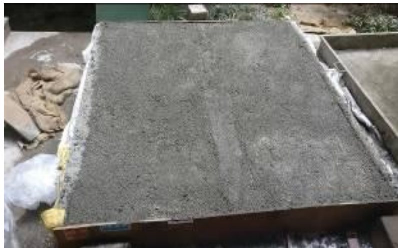
Figure 6 :- Complete casting polystyrene Concrete for (MSA) slab
