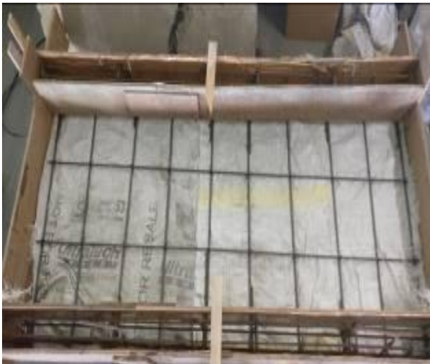
Figure 8 :- Form work of (MSB) Slab
