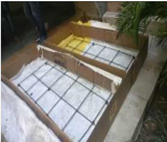
Figure 4 :- Form work of Slab
