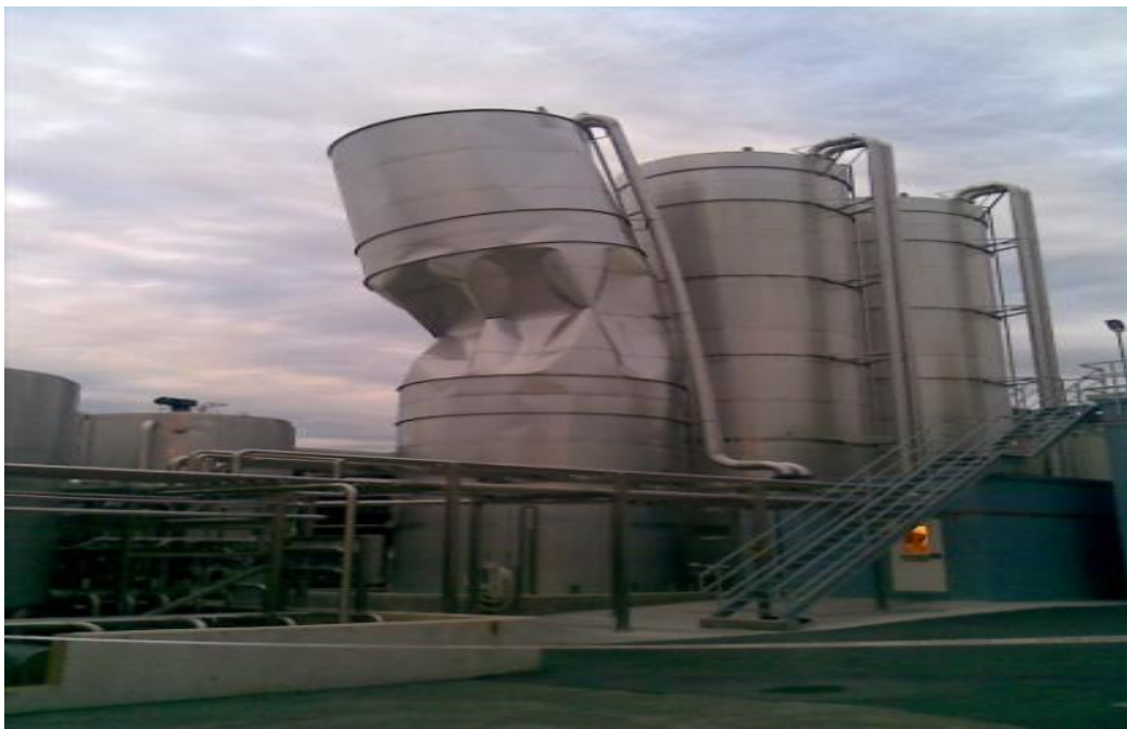
Fig 1. Buckling of silo
