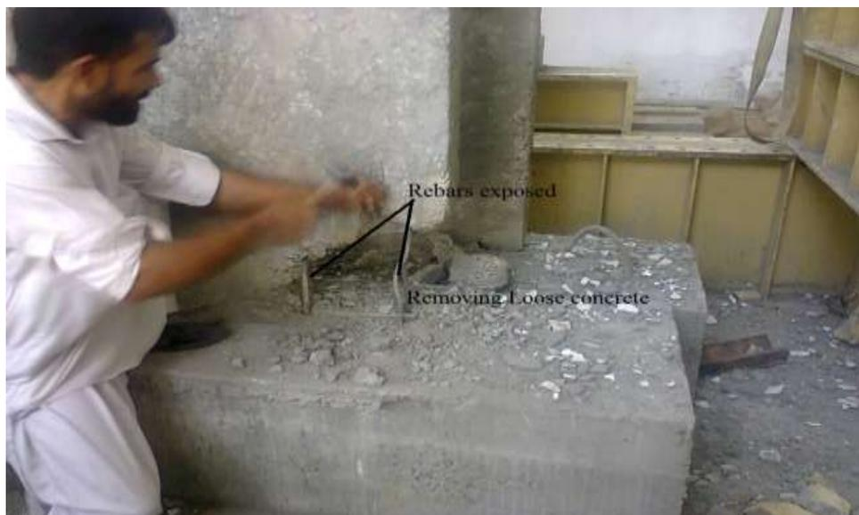
**Figure 4: Removal of loose concrete from the damaged portion of the wall after phase 1 Testing**
