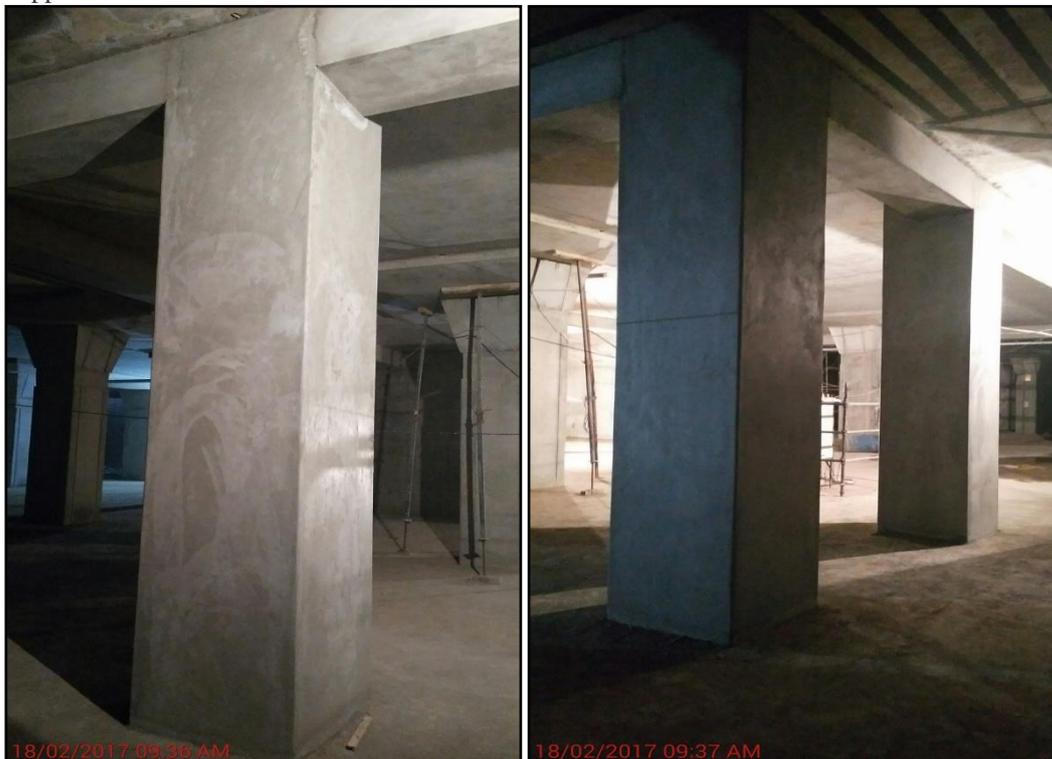
Fig.5 Cement Plaster Application
